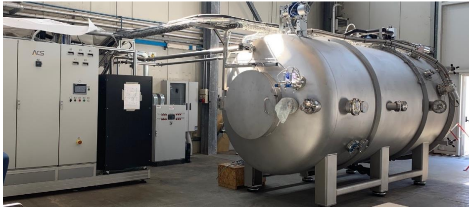
Figure 4. View of the MSVC simulator during the installation phase.
