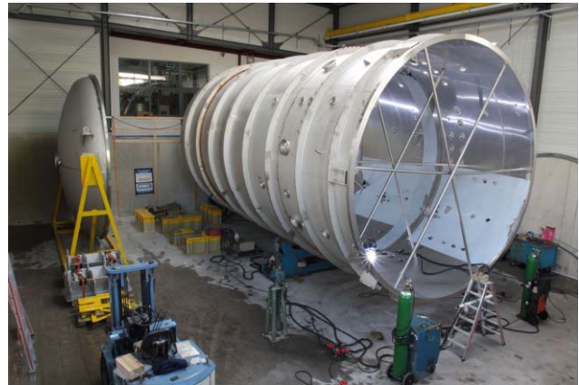
Figure 3: Assembly of the vacuum chamber segments inside the new building. The chamber segments were assembled in the factory and welded together on site at DLR.
