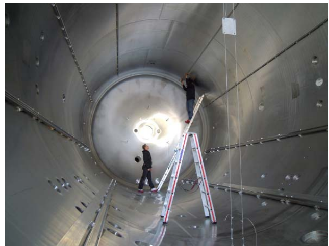
Figure 4: View into the empty STG-ET chamber during commissioning (checking of alignment and position of ports and dimensions).
