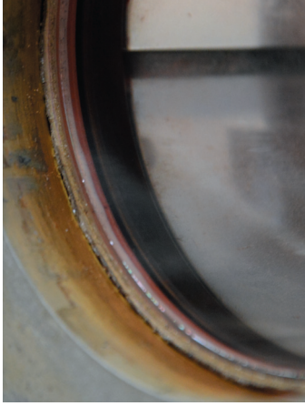
Figure 4. Damaged silicon sealing post N_2 50 I_n /min, 100 kW
