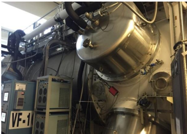
Figure 6. Side view of VF-16. The facility's controller can be seen in the bottom left of this photo, alongside 2 compressors for the 4' diameter cryopumps.
