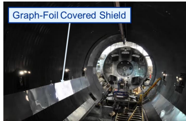
Figure 4. VF-6 during installation of Grafoil® shielding.
